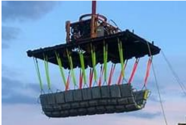
Plate 4-4: Example of Concrete Mattress Lifting
