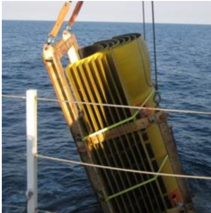
Plate 4-7: Example of GRP Cover Installation
