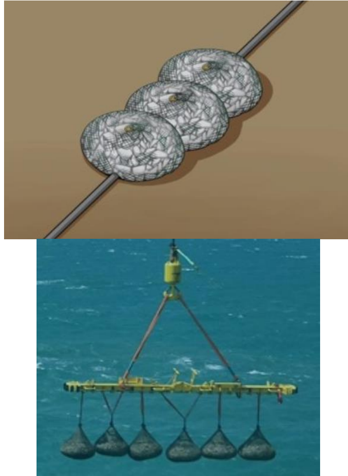
Plate 4-1: Typical Filter Unit Design and Installation
